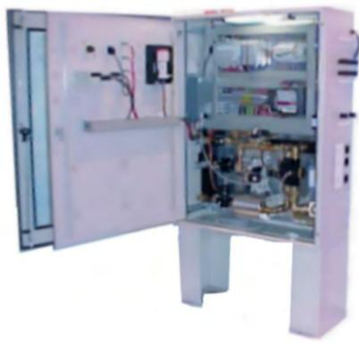
In this application a mixing panel rated at up to 180 cubic metres per hour could supply upwards of 180 welding
